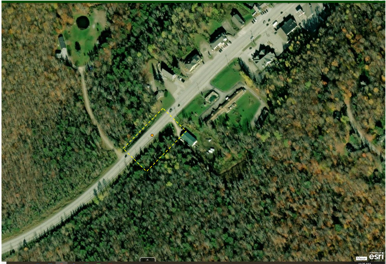
Figure 13. Survey area at Bridge 28 in Killington on US Route 4.
