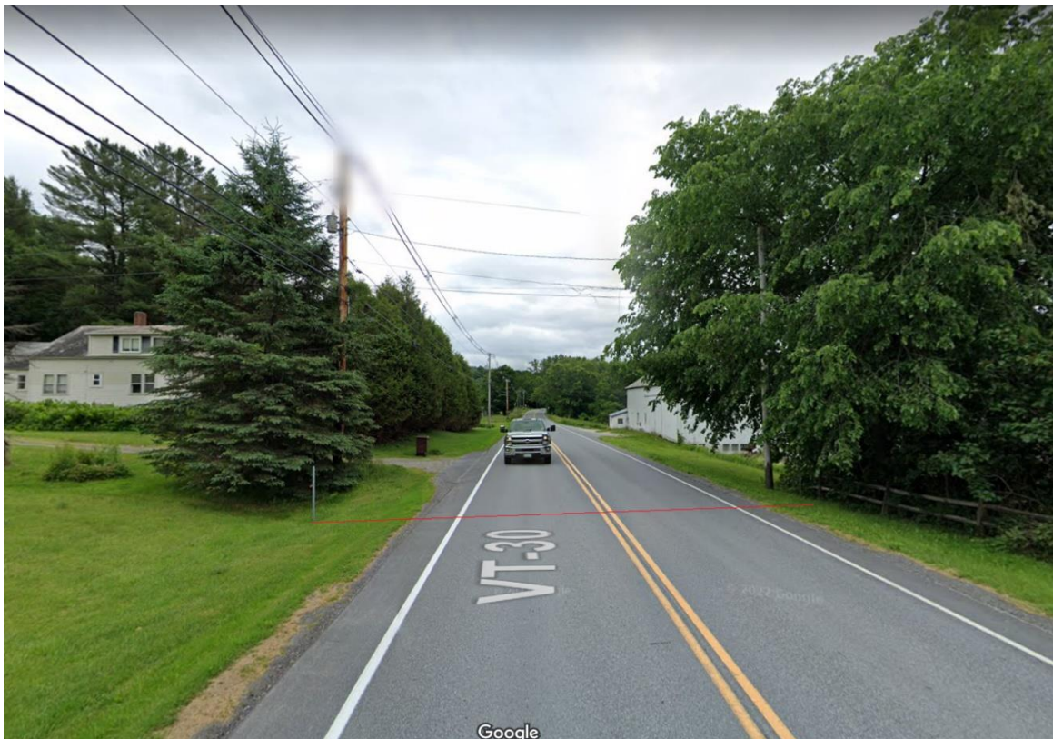
Figure 1: Overhead Utilities over the North End of the Culvert and Crossing VT-30
