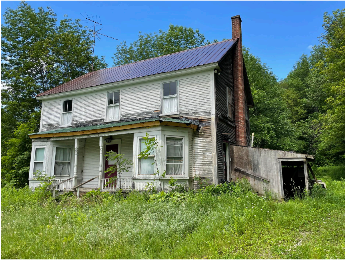
Figure 3. Vacant, deteriorated house near Bridge 36, at 1081 US Route 4 in Bridgewater. August 2022.
