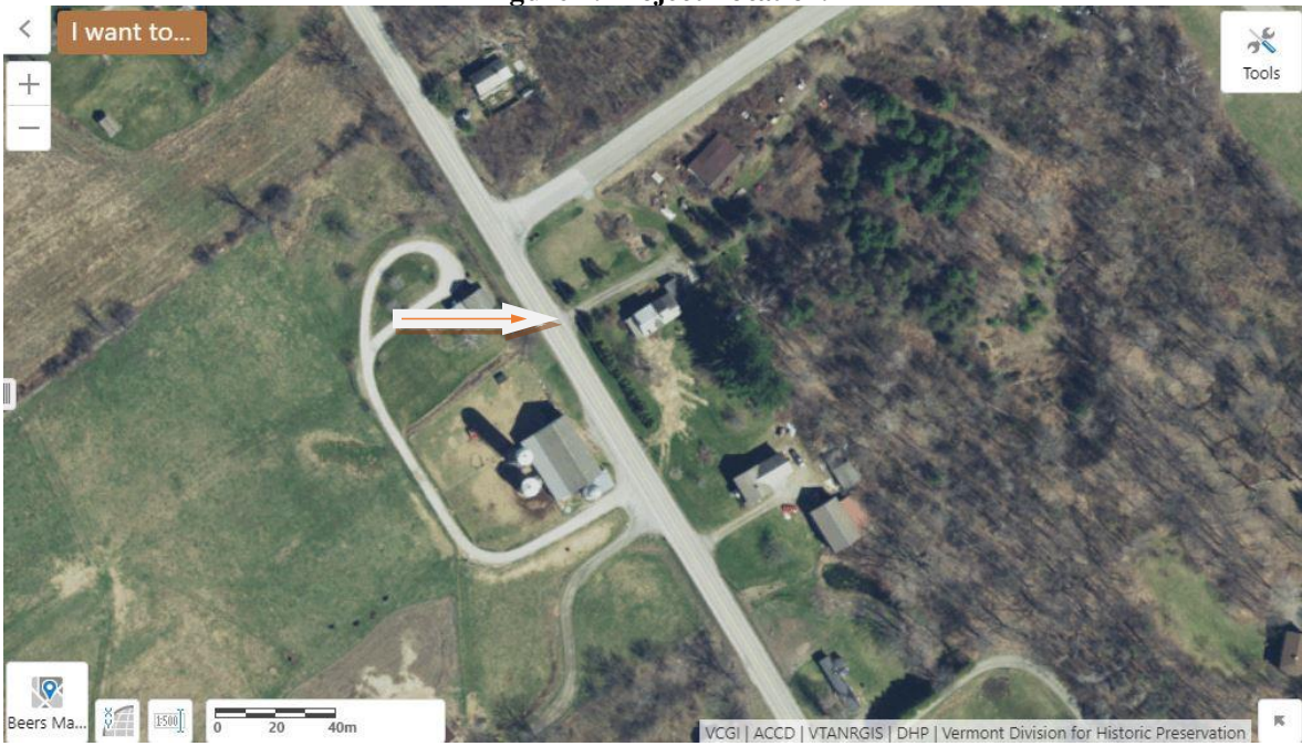
Figure 2: Project Aerial View.
