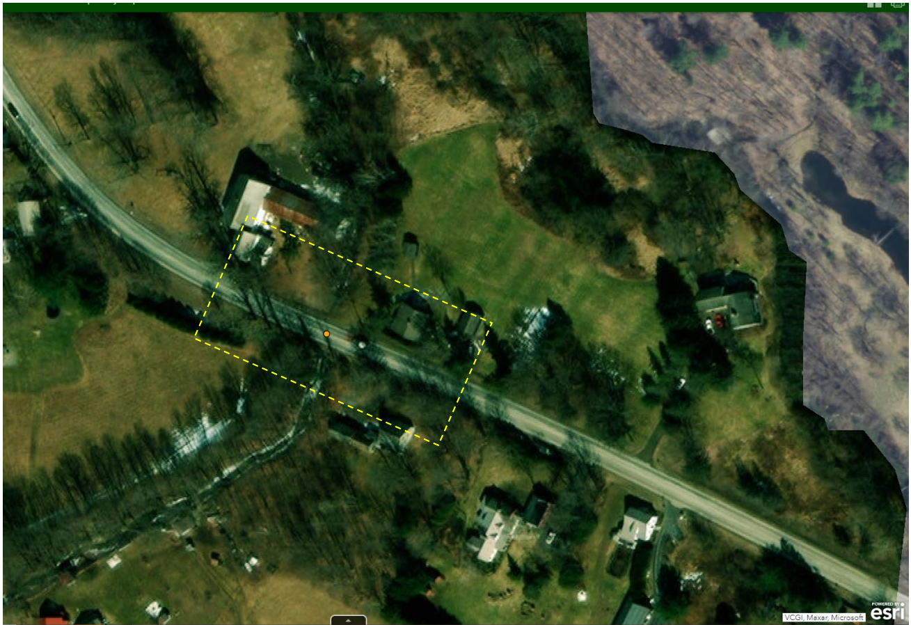
Figure 18. Survey area at Bridge 25 in Londonderry on Vermont Route 11.
